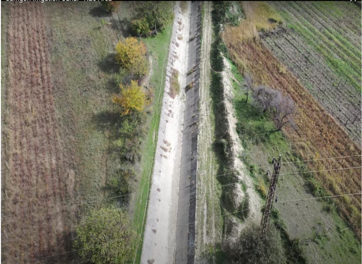
Samgori Irrigation Canal - N26 Area
