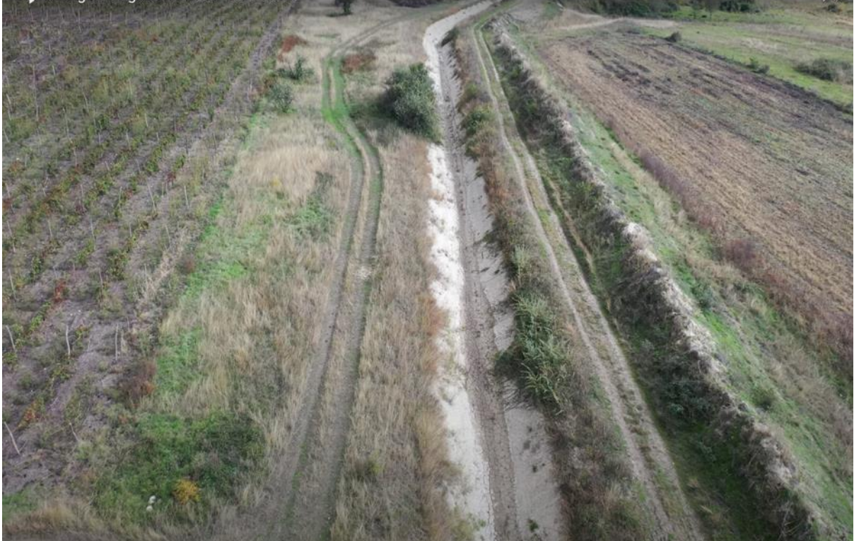
☰ Samgori Irrigation Canal - N29 Area
