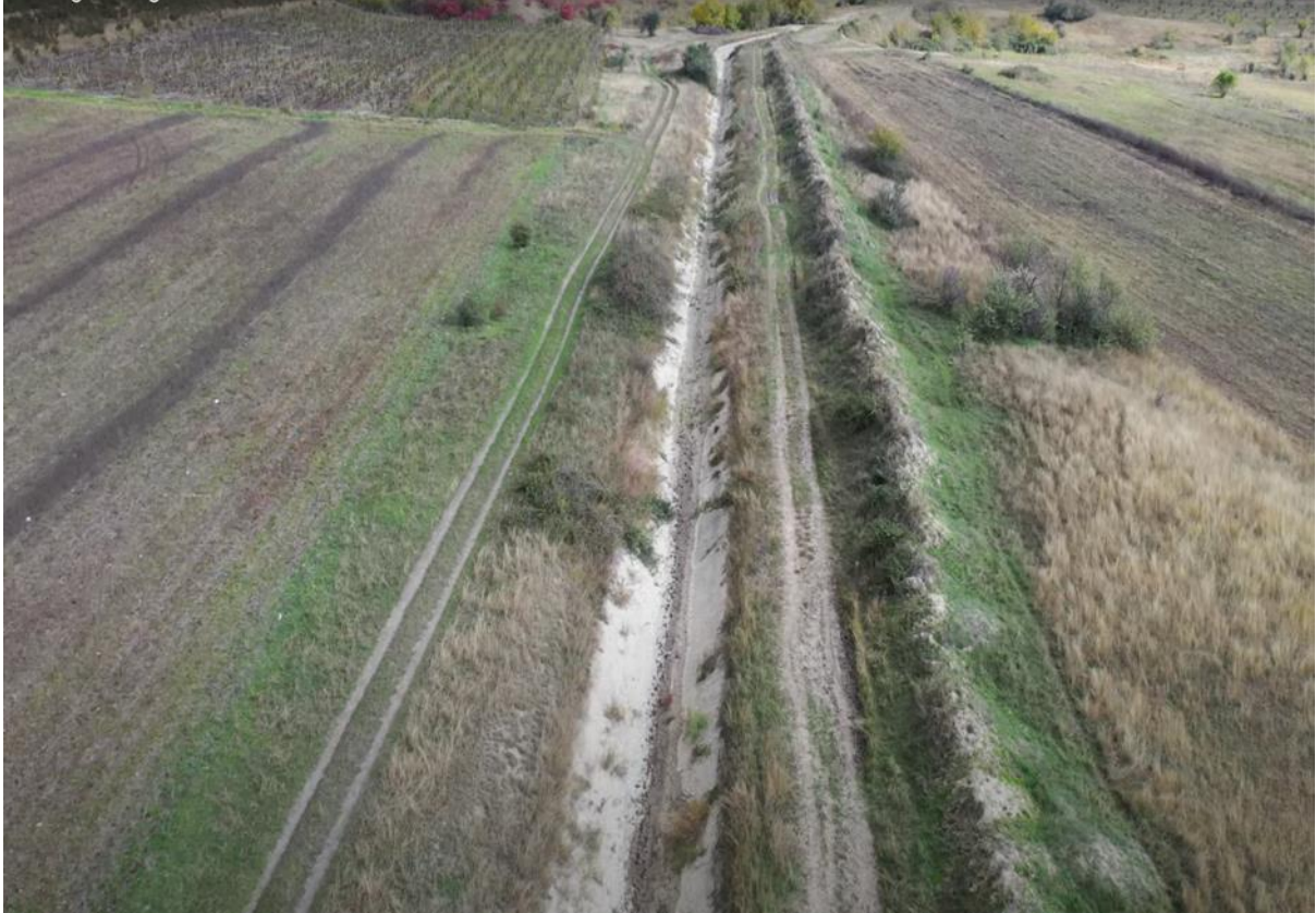
Samgori Irrigation Canal - N28 Area
