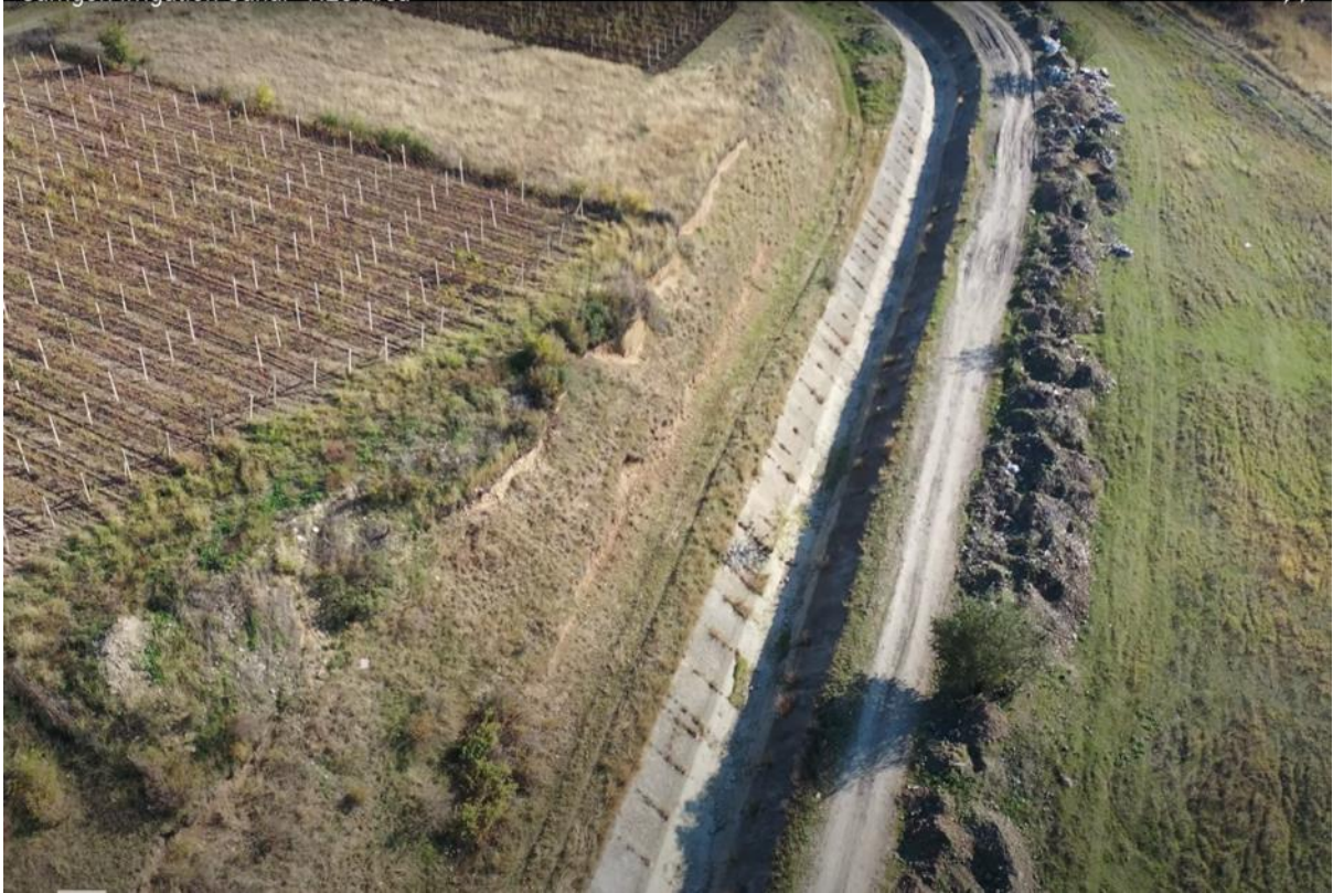
Samgori Irrigation Canal - N25 Area
