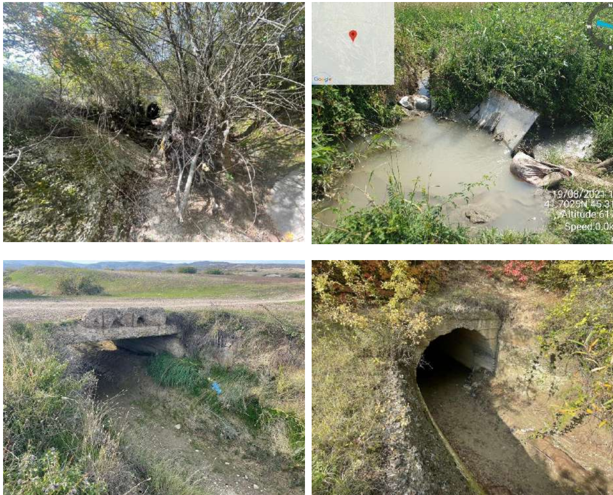
Figure 6: Condition of the Main Canal 15
