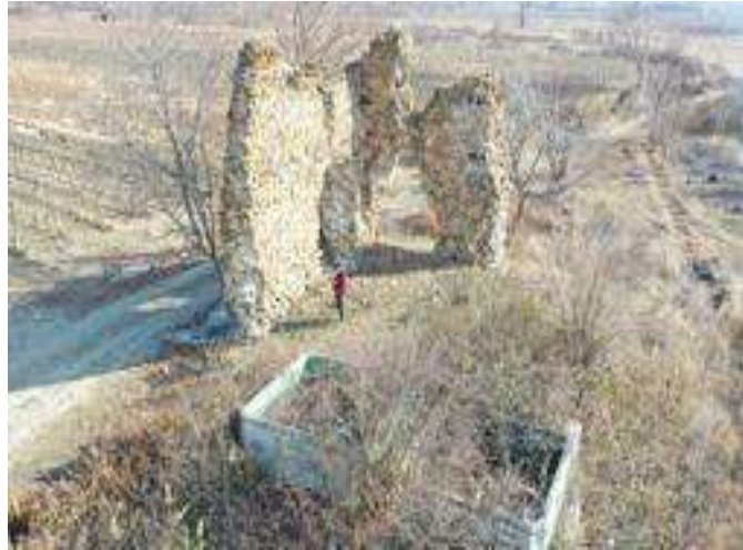
Figure 33: Nameless Tower Poor Condition
